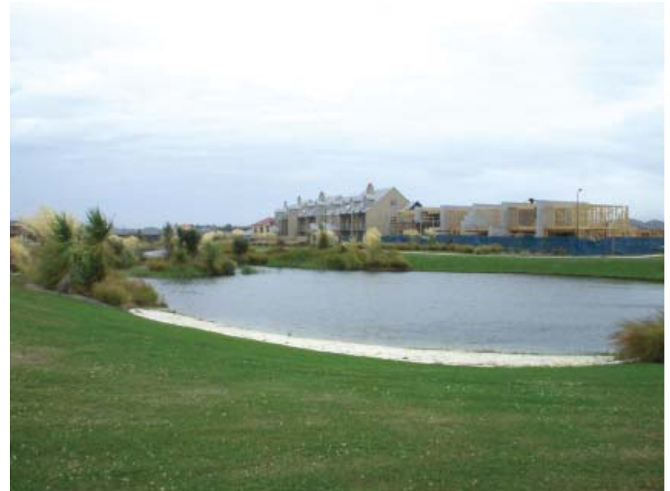
'Northwood' Housing developments like this are expected to continue in response to city growth.
