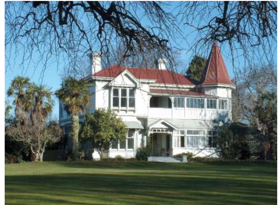
Avebury House - a recently developed community centre.
