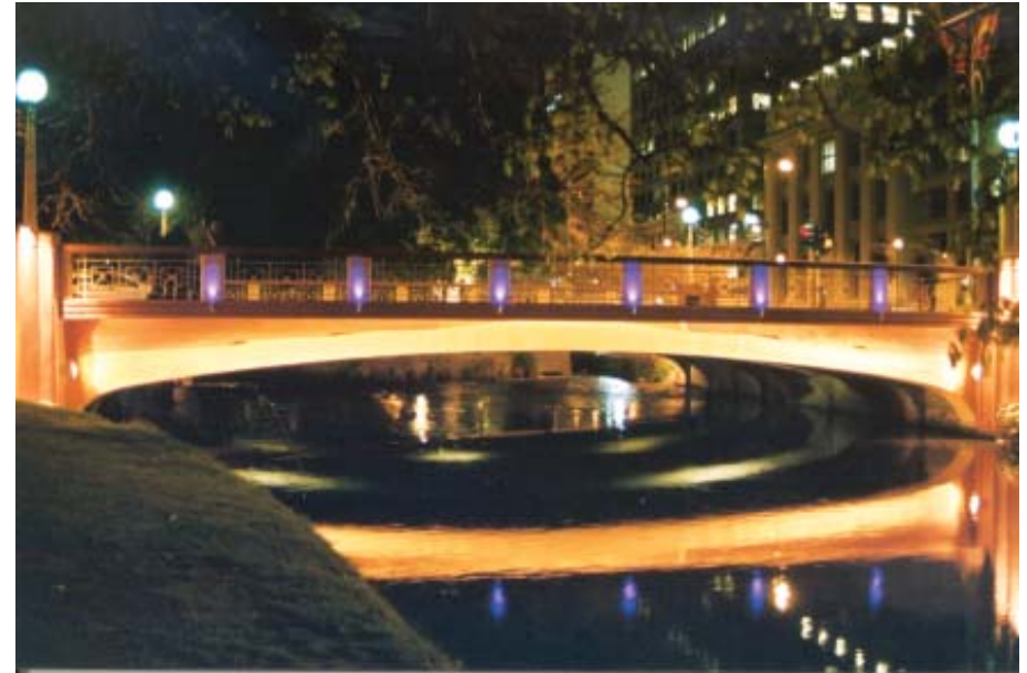
Lighting accentuates the features of the Hereford Street Bridge.
