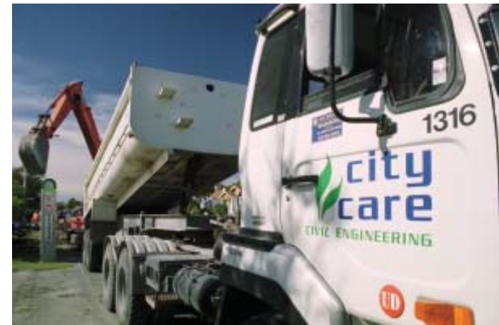
City Care replace a water sub main.
