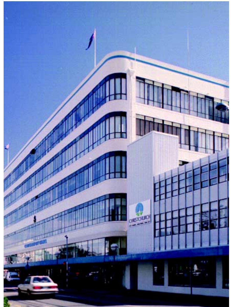
Civic Offices, 163-173 Tuam Street, Christchurch
