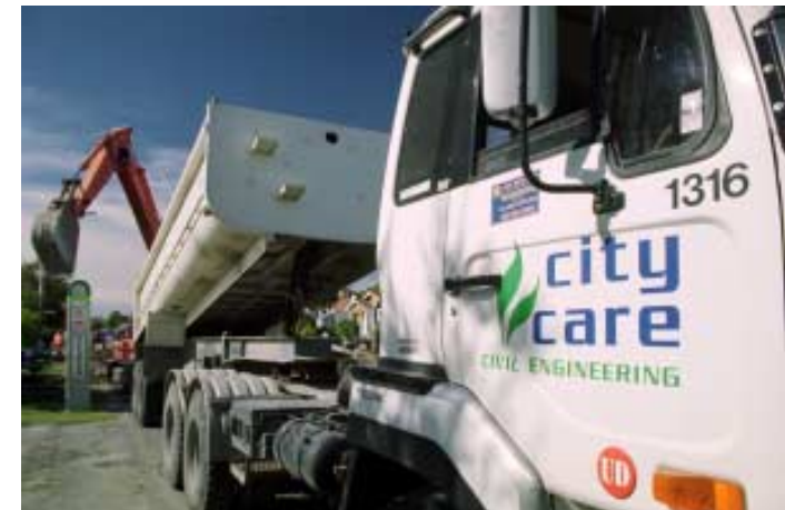
City Care replace a water sub main.
