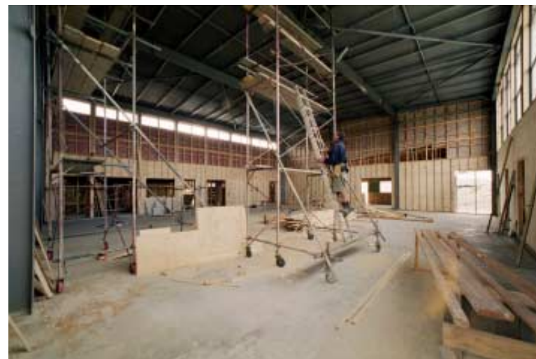
Construction work on the recently completed Parklands Community Centre.
