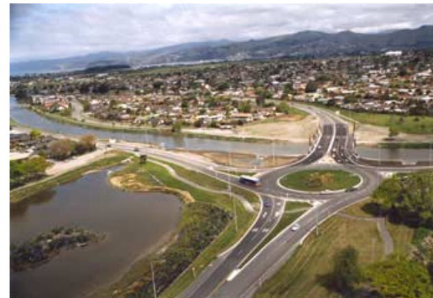
An aerial view of the recently completed Woolston Burwood Expressway.
