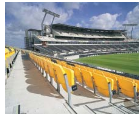
A view of the recently completed West Stand at Jade Stadium.
