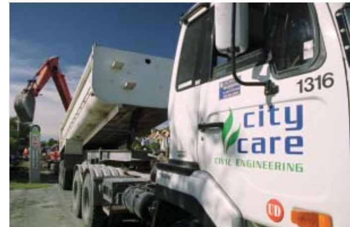
City Care replace a water sub main.
