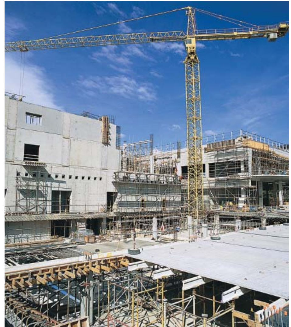
The New Christchurch Art Gallery currently under construction.
