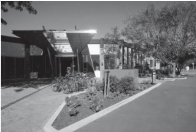
Fendalton Library / Service Centre from Jeffreys Road
