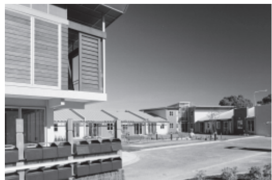
The recently completed Council housing complex in Goulding Avenue / Main South Road, Hornby
