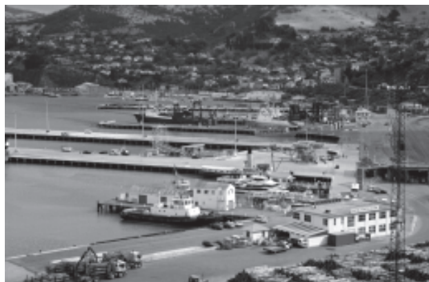
The Lyttelton Port Company facilities
