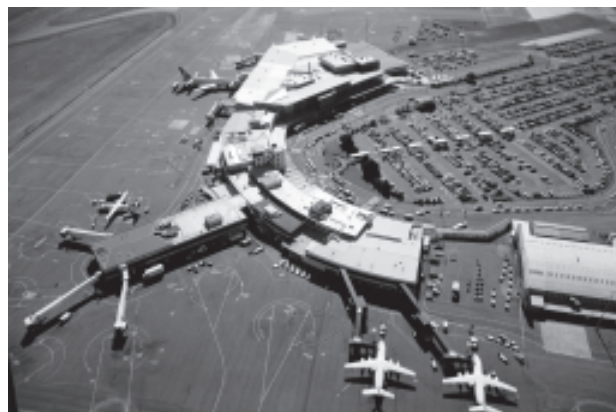
Christchurch International Airport Company terminal facilities from the air
