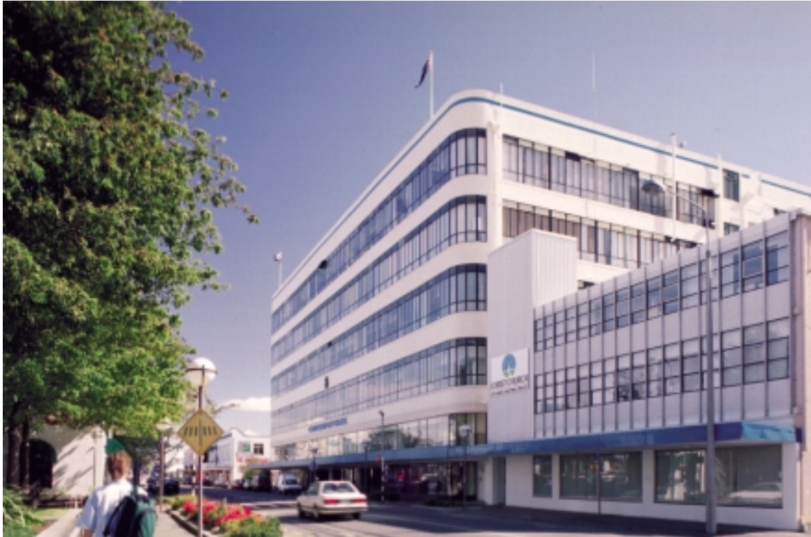
Civic Offices 163 Tuam Street, Christchurch
