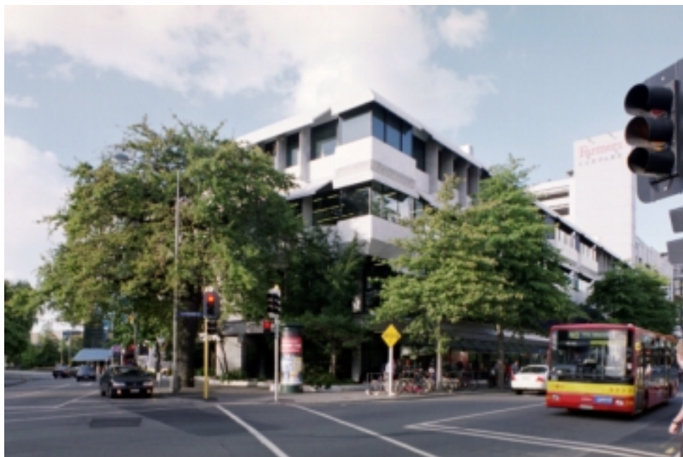
The Central Library from the Gloucester Street / Oxford Terrace Corner
