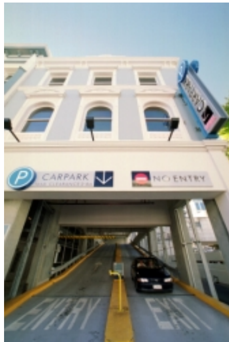
The entrance and exit to the new Bus Exchange Car Park
