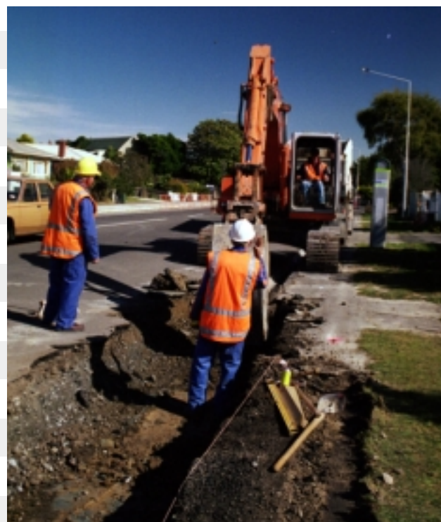
Kerb and channel work being undertaken in Woodham Road
