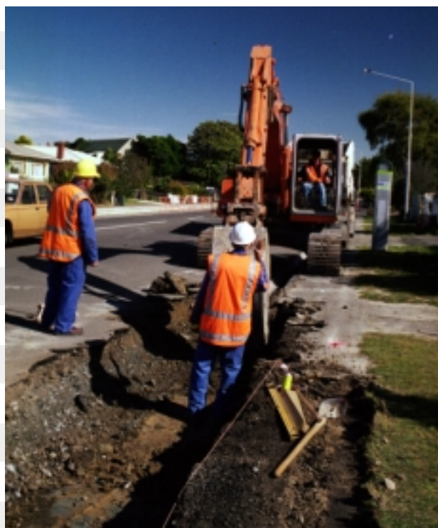
Kerb and channel work being undertaken in Woodham Road
